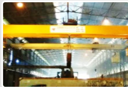
Coil handling crane
