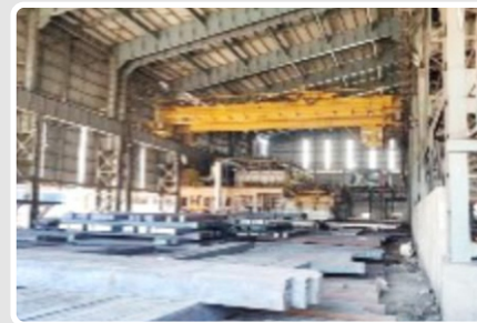
Raised Girder crane
