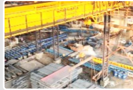
Billet handling crane
