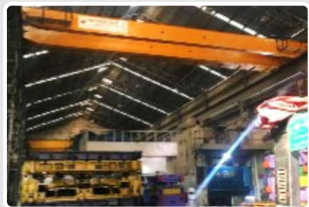
Dies handling crane
