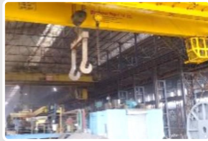
Bar handling crane
