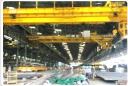
Bar handling crane
